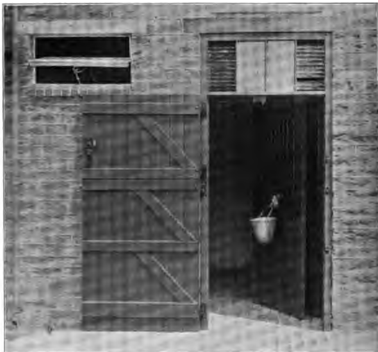
Fig. 27. Water bucket fixed to door of box.
